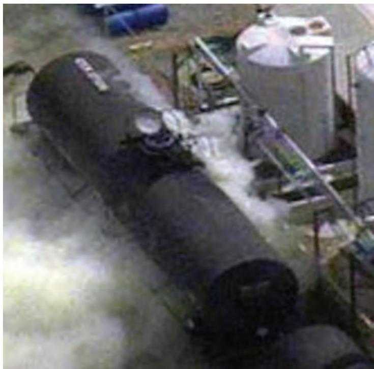
**A chlorine repacking plant receives 4 railcars contained nearly 250,000 lbs of chlorine to be repacked into cylinders and other distribution. After 59 days, a hose wrongfully identified as a chlorine hose catastrophically failed spilling 48,000 pounds of Chlorine over 3 ½ hours. The root cause in addition to the hose failure, is that backup systems (ESD'S) as well as excess flow valves (EFV's) failed to work**
